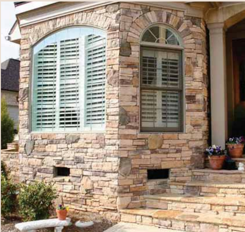
80% Seneca Dry Stack with 20% Pennsylvania Fieldstone
